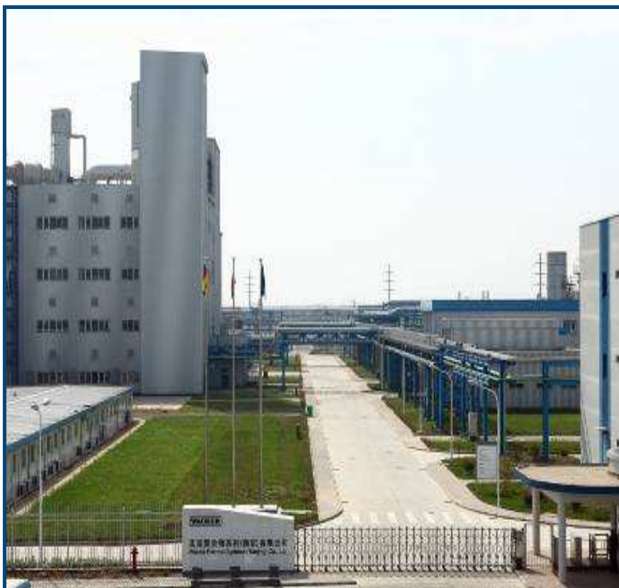
Polymers Site in Nanjing (China)
