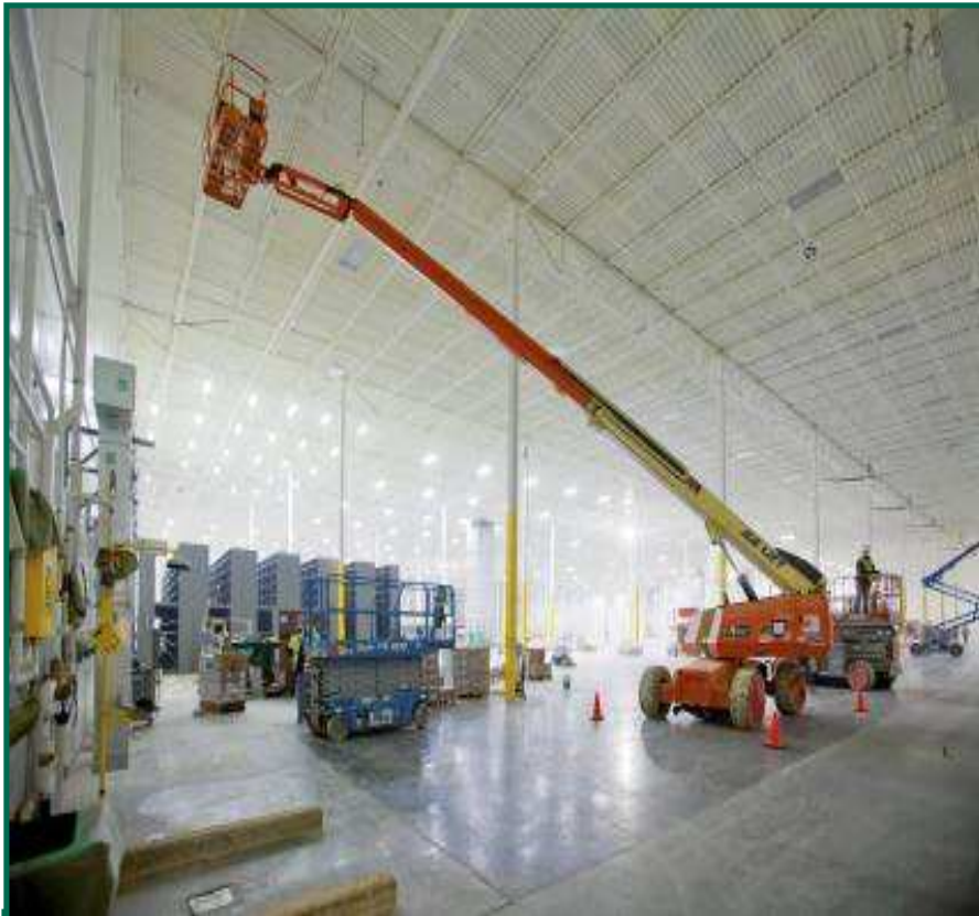
POLY 11: Production hall in Charleston, TN
